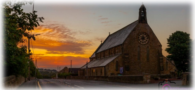
St Ives Church, Leadgate
