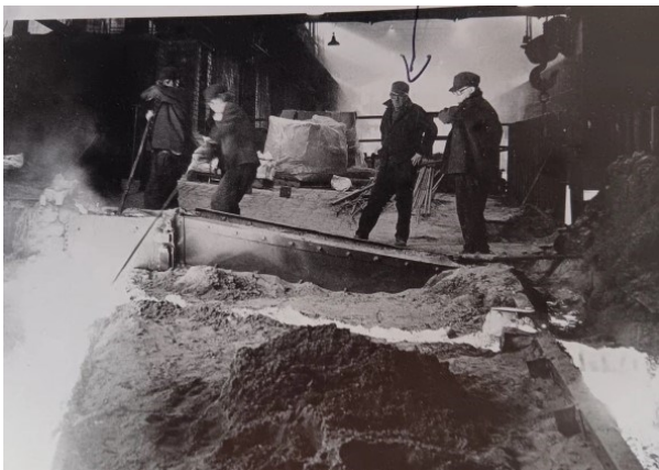
John Hegarty Jnr 2nd Right At the black furnace, Consett ironworks 1978
